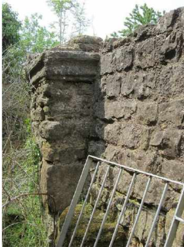
Figure Eight The North Gate: An Internal Impost
