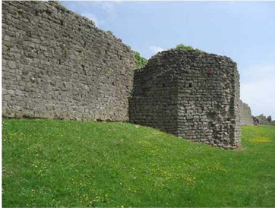
Figure Two South Wall with Bastion looking East
